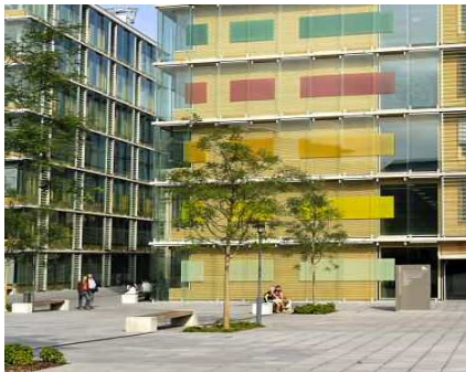
University of Applied Sciences Frankfurt am Main, Germany
